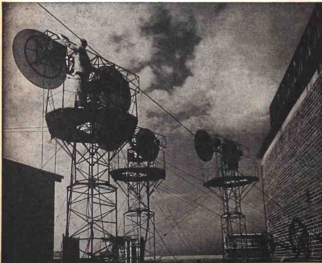
Rear view of three parabolic antennas on roof of the Telephone Building, New York City.
